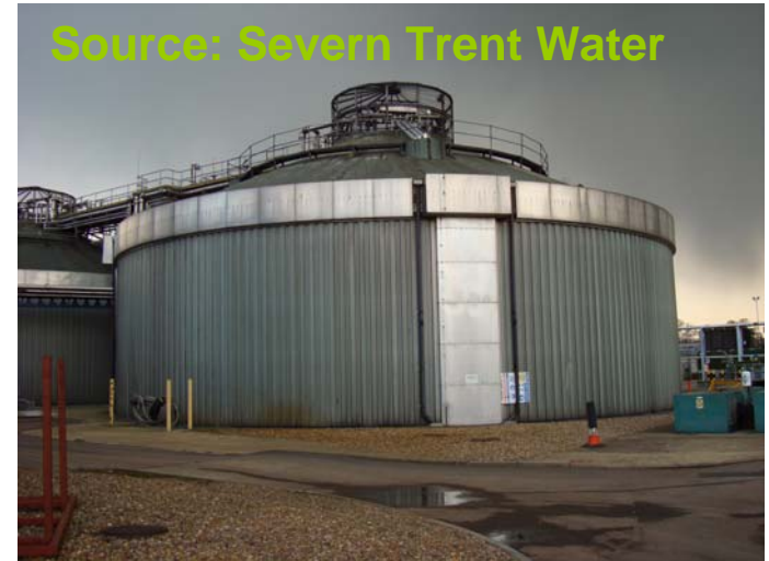
Typical Sewage Works Digestion Plants
